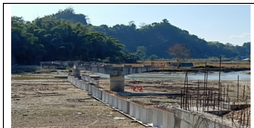
Bridge over Pachin river as on Dec 2019
