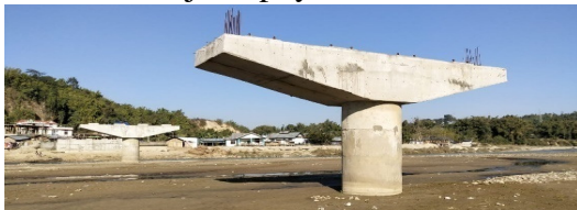
Bridge over Pachin River as on July 2018
